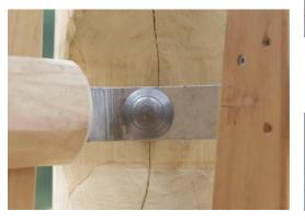
The hardware is made of stainless steel or galvanized steel to ensure durable connections with a high corrosion resistance.
